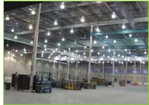
Before Metrolight 400w magnetic HID ballasts
