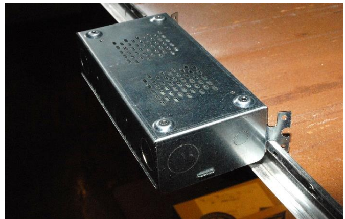
Mounted to T-Bar using the integral T-Wings
